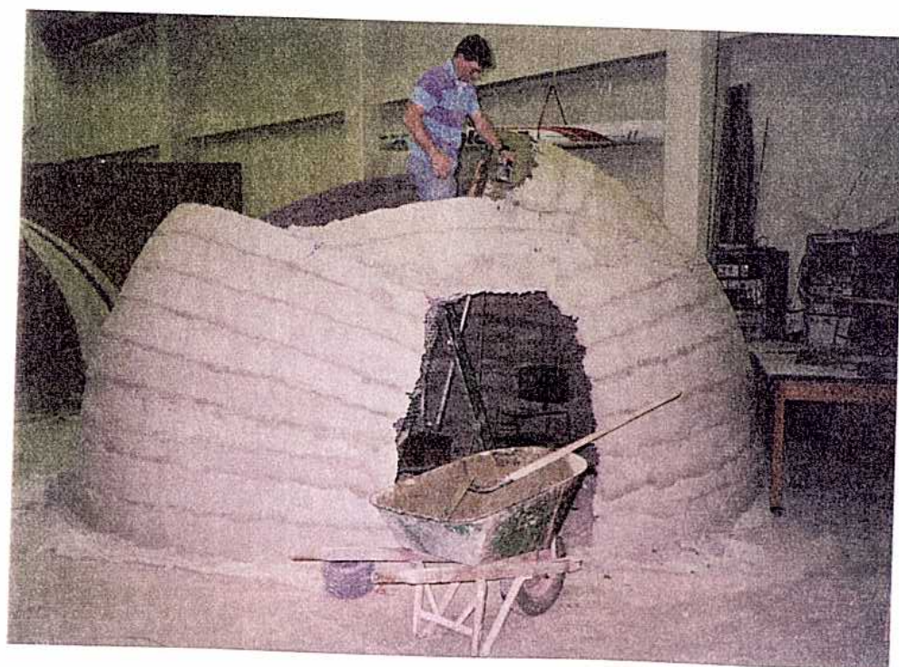
Figure 18. It is now easier to spread out the concrete from inside.
