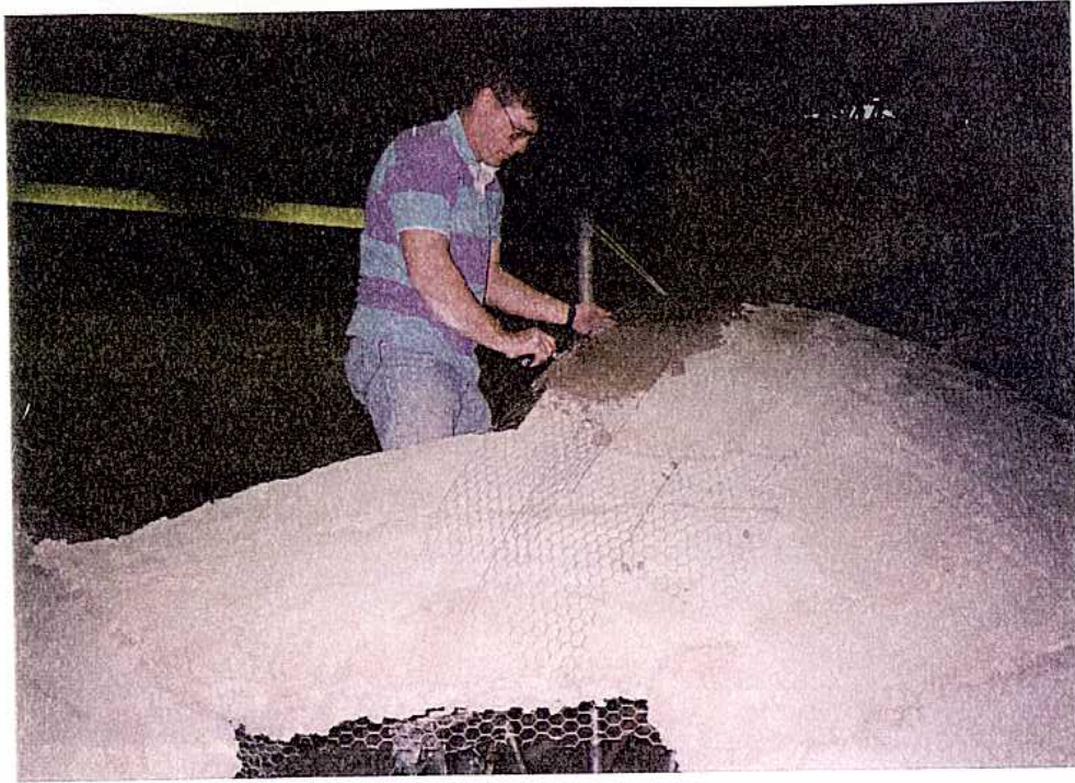
Figure 21. As the layers are going up, generous portions of wire fabric are overlapped and left to bond the future exterior layer.
