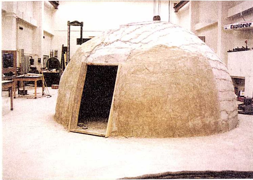
Figure 29. Front of dome after partial second layer of concrete has been added.
