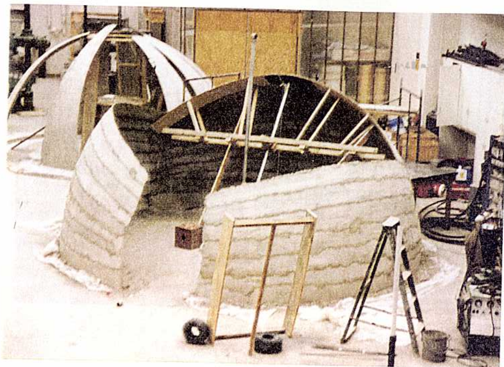
Figure 17. A great view of the back of the dome and how the form is "shored up."
