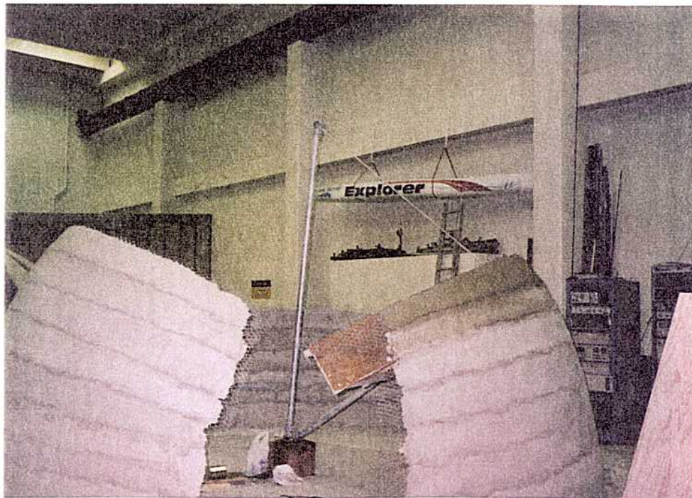
Figure 16. Last lift before crossing over the door opening.
