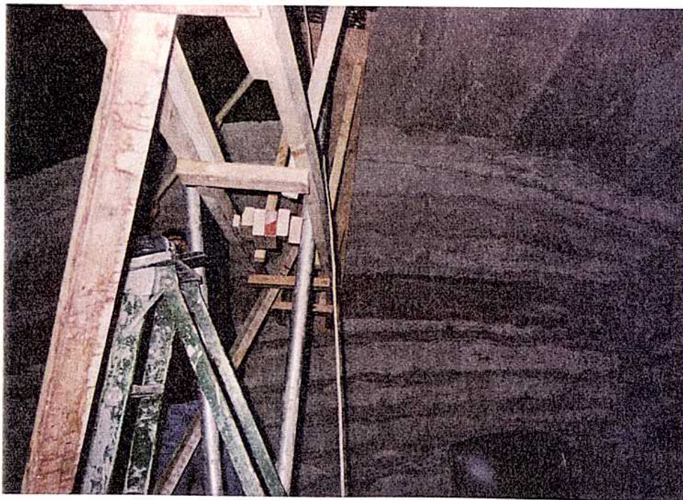
Figure 20. Last lift on the right side of dome. At this point it is easier to shovel the concrete from the inside.
