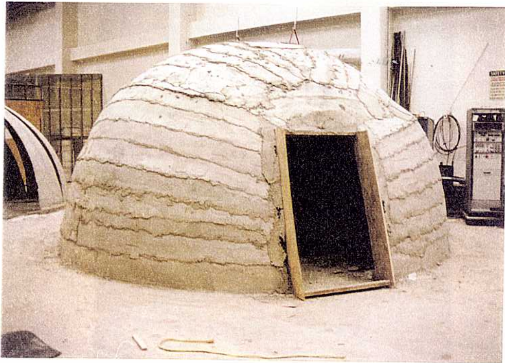
Figure 23. Exterior of finished dome after first layers of concrete. It looks very “igloo” like.
