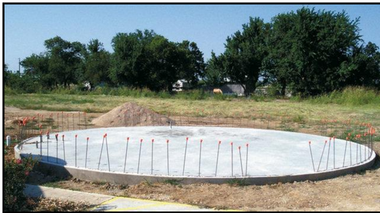
Figure 3: Typical cement foundation for a Monolithic Dome. 13
