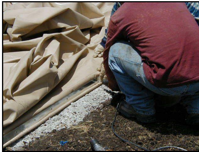
Figure 4: Airform being attached to the cement foundation. 14
