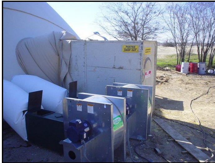
Figure 5: Airlock entrance and fan blowers properly installed. 15
