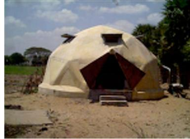
Figure 6.4: Ferrocement Geodesic Dome in Sri Lanka [geocities, 2006]
