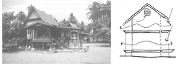
Figure 7.5: The steeply pitched roof of a Malay house, the roof utilizes gable vents to promote cooling. This is illustrated by a sketch of the design approach. [Hyde, 2000]
