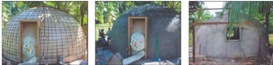
Figure 4.23: Construction of an 'Ecoshell' [Hennik, 2005]
