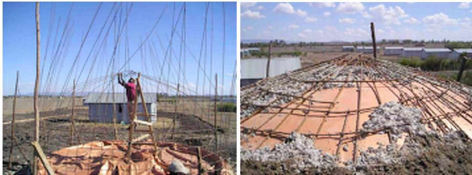
Figure 11.1: The airform did not reach the rebar cage in Ruia, Kenia [Spit]
