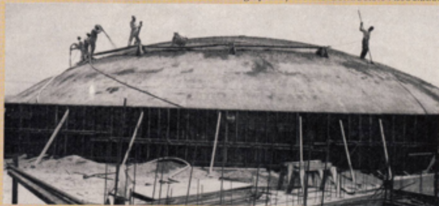
Guniting operation under way on the dome of White Memorial Seventh-Day Adventist Church. Height of dome above the floor is 70 ft; the diameter is 107 ft
