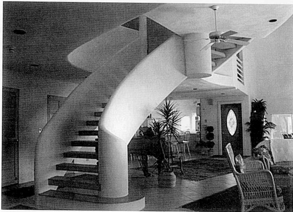
Figure 30 One view of the interior of the "Eye of the Storm." Ceilings are suspended from the roof of the dome. Note also the curved walls and staircase.
