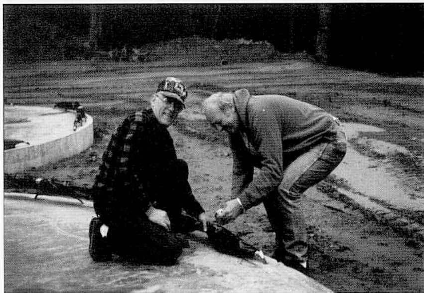
Figure 10c Folded rebars wrapped to avoid cutting into the skin.
