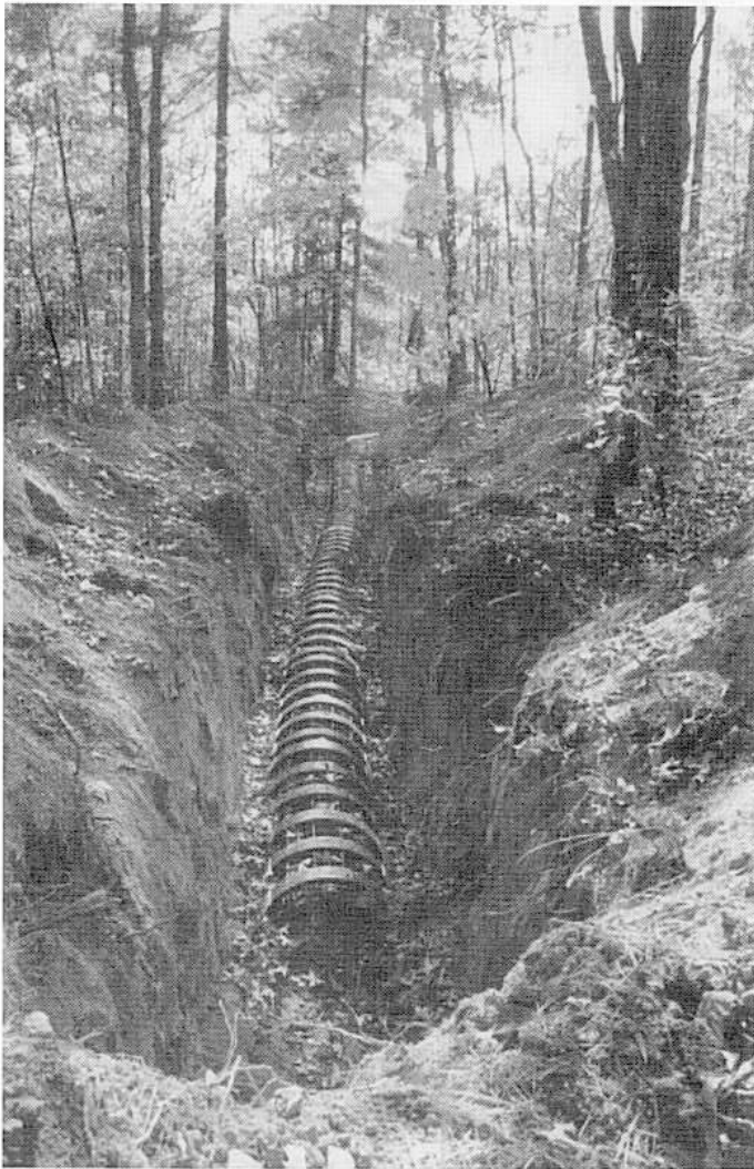
Figure 54 The latest in Septic systems Technology (the infiltrator system).
