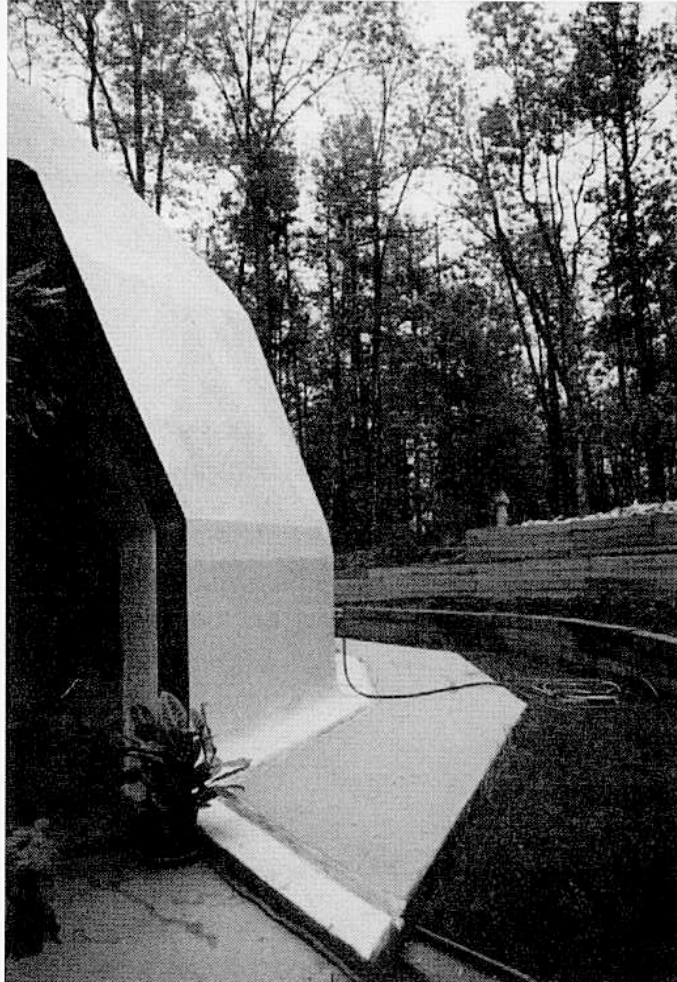
Figure 44 Footing around a geodesic dome.
