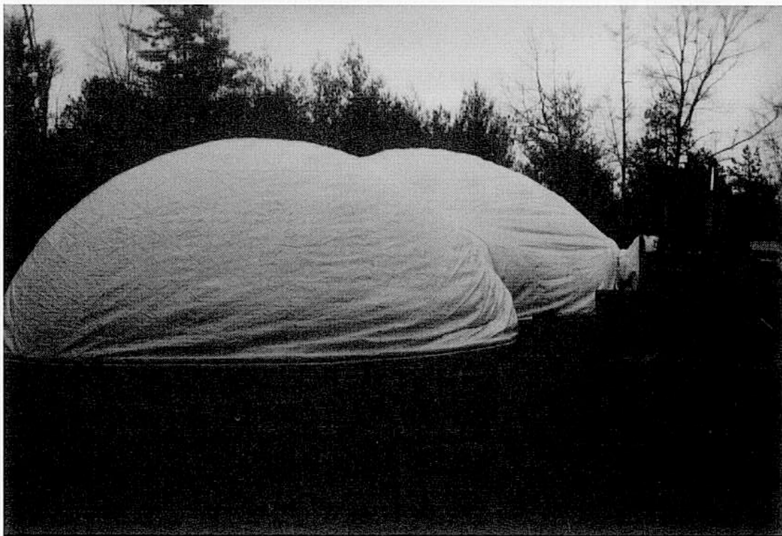
Figure 13a Early stage of inflating the dome skin.
