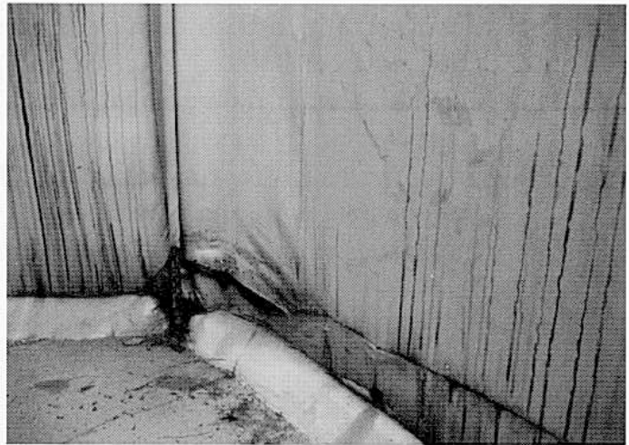
Figure 42 Pulling away of the skin from tension on the patch.
