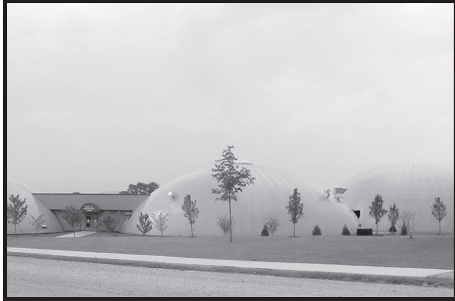
Figure 2.5 — During the 2007-2008 winter, Caledonia, Missouri experienced ice and wind storms that covered their area with two to three inches of ice and left people without power for up to two weeks. Superintendent Steve Yount said that the domes were unaffected by the cold, and, although they were without power, the domes retained their heat, so people spent their days warming up in the Monolithic Domes. The community wants their domes certified by the Red Cross as a designated disaster shelter and is looking into grants that would finance a generator.
