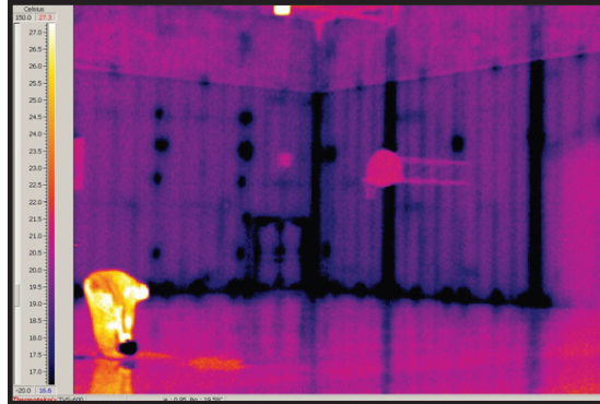
Figure 2.15 — Internal image of a metal gymnasium near by. Note the bright colors of the student and the below-zero colors of the exterior walls.
