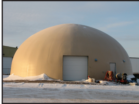
Figure 2.9 — Heated Monolithic Dome shop in Saskatoon, Saskatchewan, Canada. The outside temperature at this time was 13 degrees Fahrenheit below zero (-25C). This is a standard color photograph taken by a standard camera. Note the metal buildings in the background.
